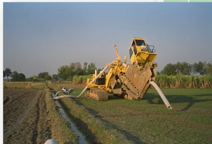
Agricultural Drainage Trencher for installation of PVC lateral and collector pipes
