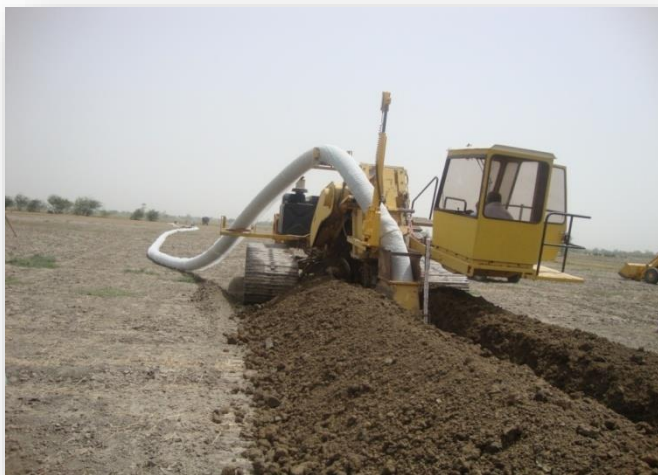
Installation of collector & lateral pipes
