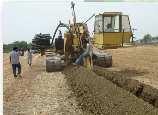
Installation of collector & lateral pipes
